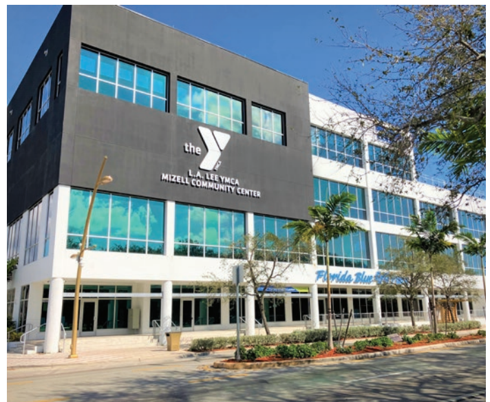
Completion of the L.A. Lee YMCA/Mizell Community Center
