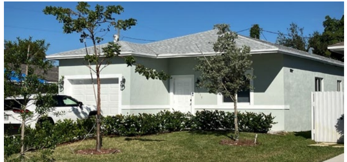
Scattered Site Infill Housing Dorsey Riverbend Neighborhood - Fort Lauderdale CDC
