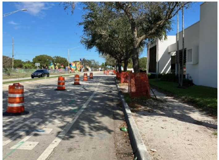
NE 4th Avenue Improvements under Construction
