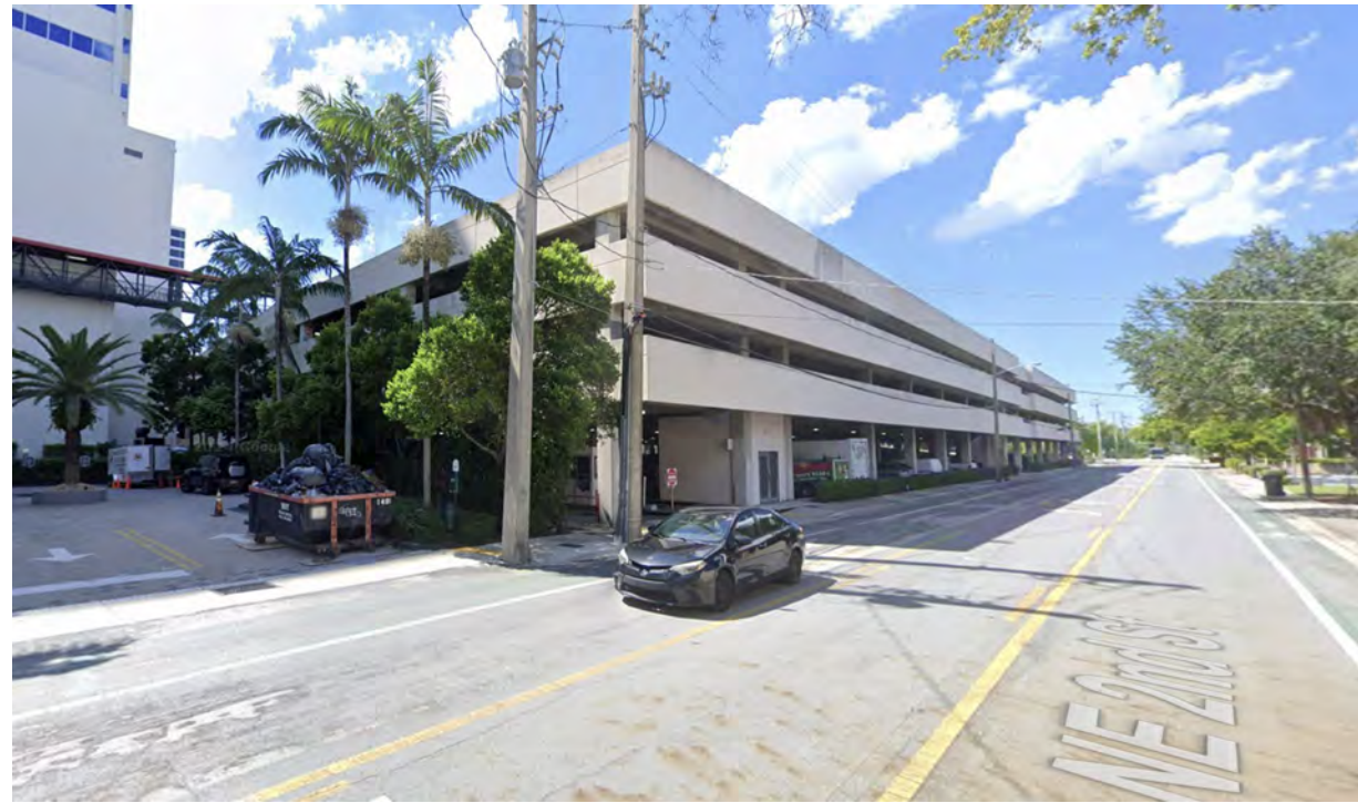
7 VIEW OF GARAGE TO SOUTH OF SITE Scale: 1/16" = 1'-0"
