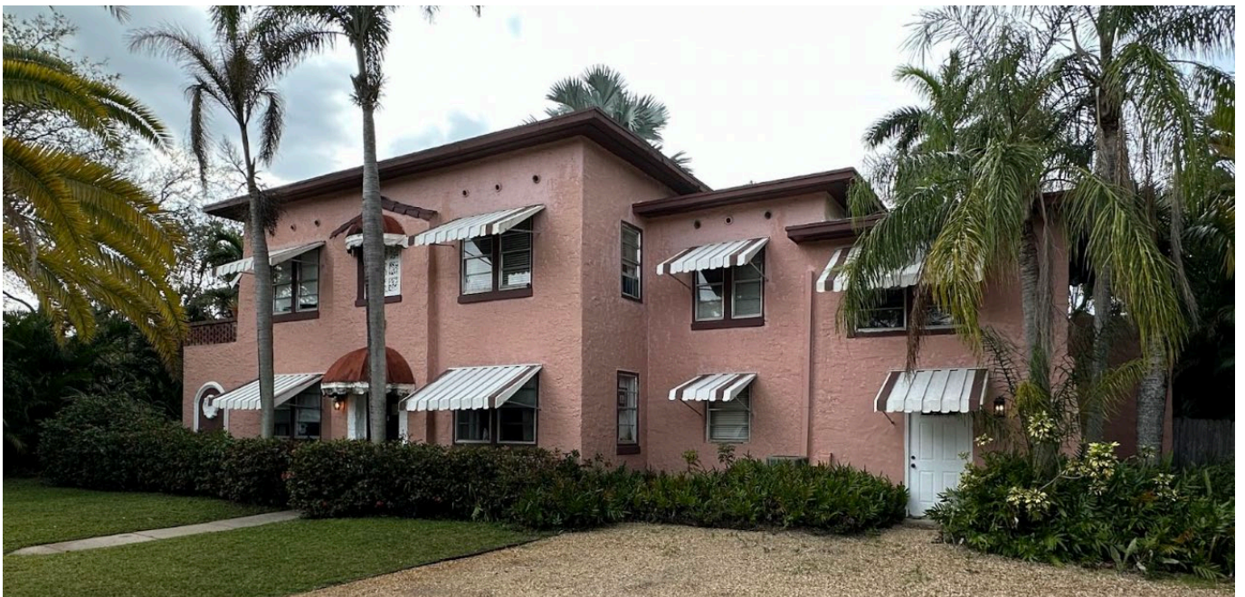
Image: 1625 NE 1st Avenue, February 2024
