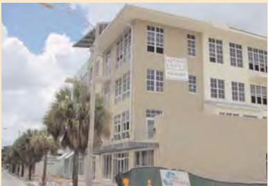
[Figure 3.30] Examples of recent projects that exhibit contemporary architectural styles that are appropriate to South Florida traditions.
