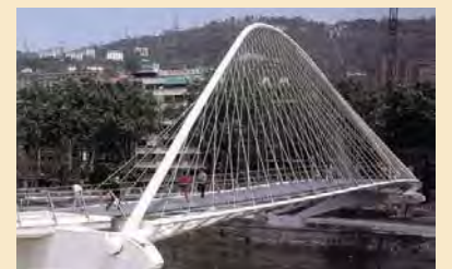
Pedestrian Bridge in Bilbao, Spain
