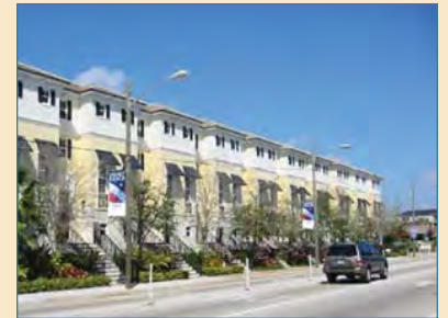
[Figure 4.122] Delray Beach - Each unit has separate entrance - Garden areas and steps enhance privacy
