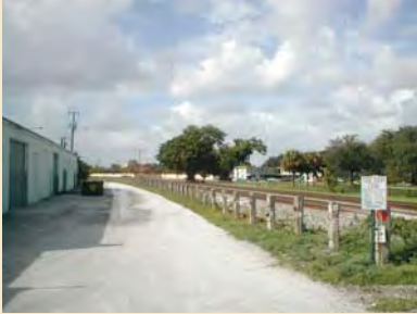
[Figure 3.51] Existing FEC Rail line.
