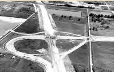
[Figure 2.8] Florida Turnpike under construction.
