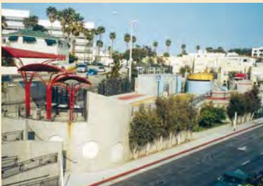
[Figure 3.38] The Santa Monica Urban Runoff Recycling Facility, Santa Monica, CA. It treats stormwater runoff for use irrigating City parks, streetscapes, and greywater for City-owned buildings, reducing pollution of the Santa Monica Bay.
