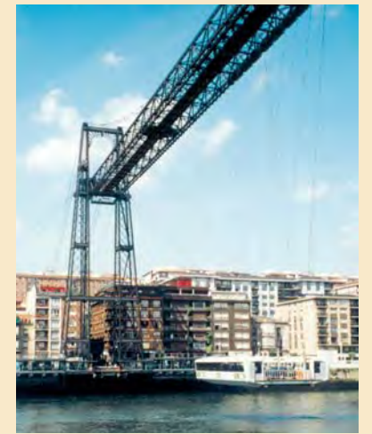
[Figure 3.14] Suspended movable pedestrian cab in Bilbao, Spain.
