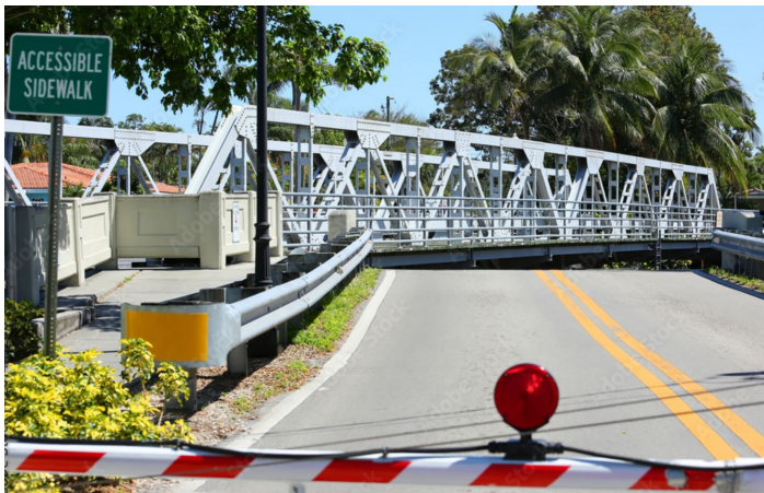
Photo: Swing Bridge
