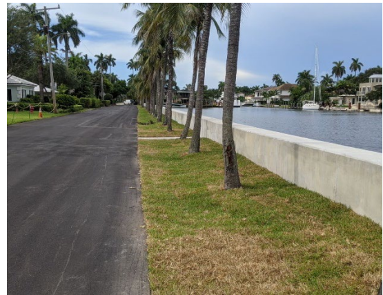
Isles of Palms Seawall after improvements
