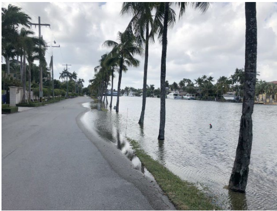
Isles of Palms Seawall before improvements
