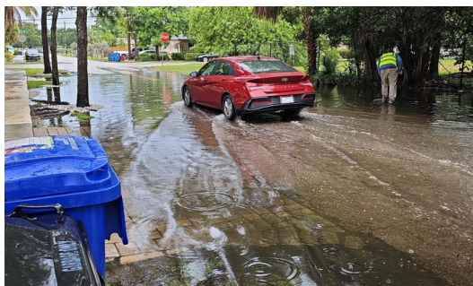
Wet Weather Site Visits
