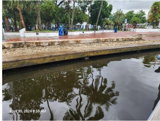
Figure 2.5.6 Wall Elevations Below Required Ordinance (WALL 41)
