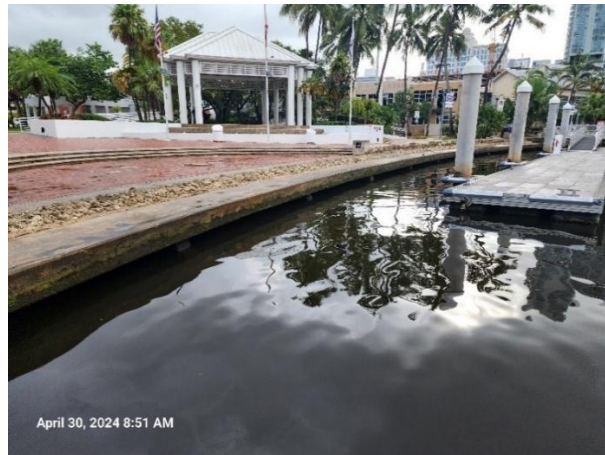
Figure 2.6.2 Wall Supporting Parking and Structure Facilities (WALL 41)
